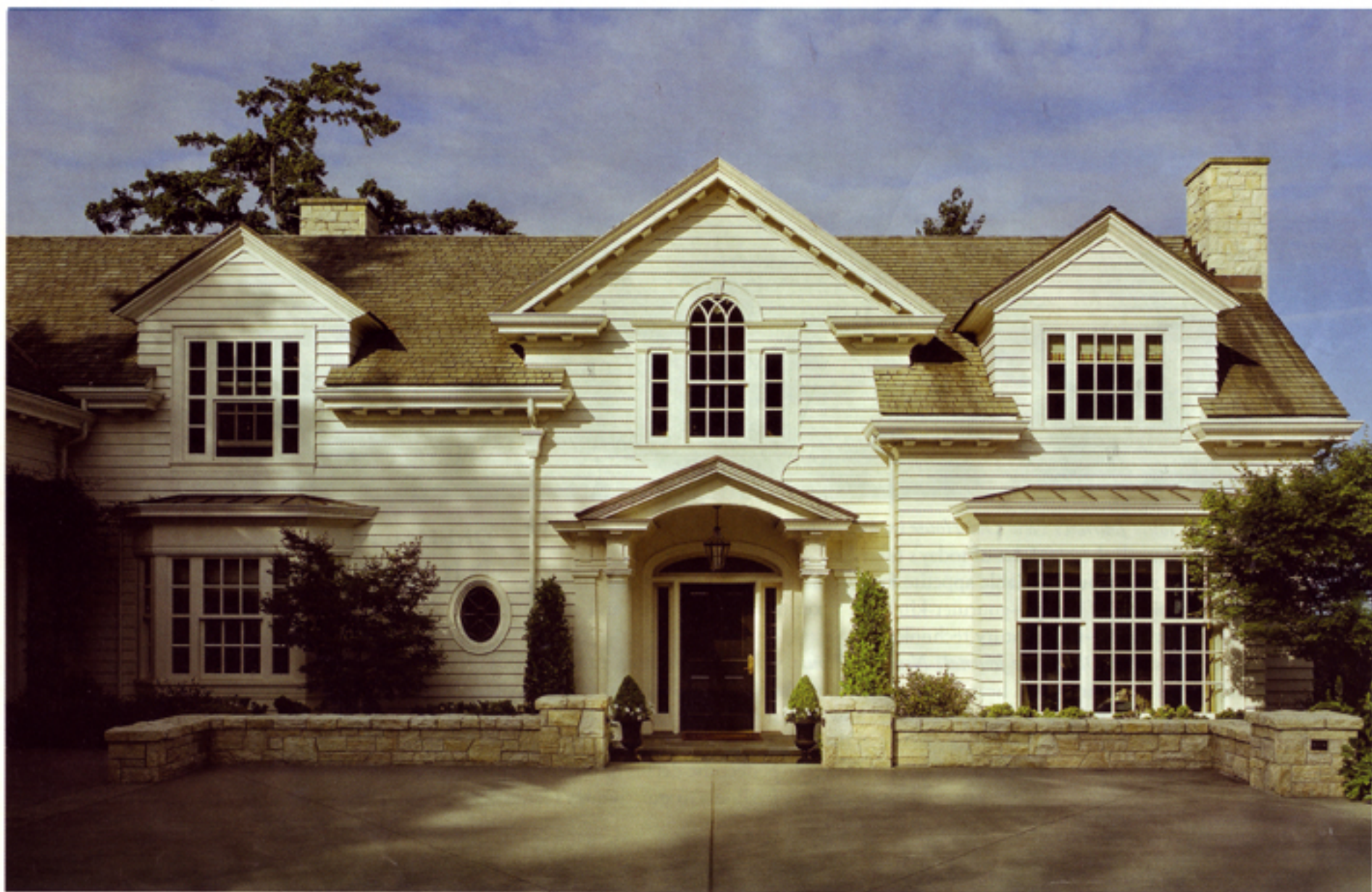
Seattle, WA-based Sullivan Conard Architects used painted cedar clapboard and shingle for the exterior of this house in Medina, WA, to convey the Classical architecture of New England. Photo: Benjamin Benschneider
