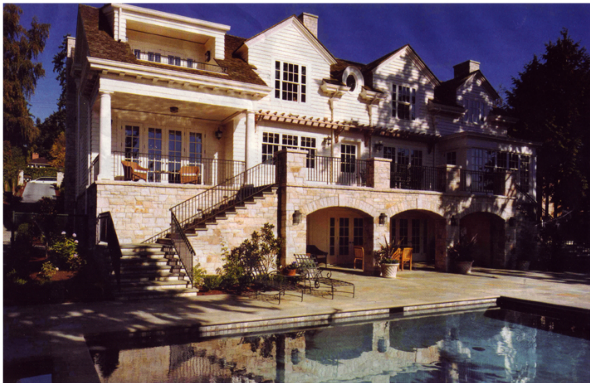
A natural terrace in the landscape was reinforced to create the pool terrace and negotiate a steep incline at the rear of the site. All photos by Art Grice unless otherwise noted
